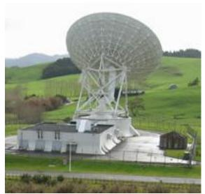
variation of 1 mm deviation of surface accuracy. It would be usable up to 22 GHz with some reduction of gain. Both dishes have switchable left / right hand circular polarisation.
