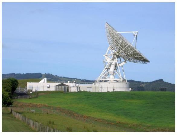
location of known point sources in the sky. Fortunately the analysis of this data is straight forward. This process is redone quarterly to confirm accuracy. Following this calibration the tracking accuracy is about +0.0001°. The 12 m dish is
